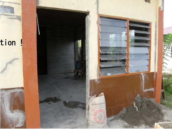
Rough surface shall be made on the oil paint surface of Block wall
